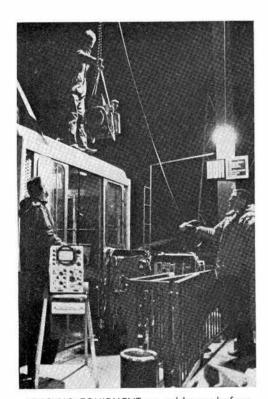
LOADING EQUIPMENT on cable car before sunrise, Sandians prepare for terrain measurement project. The car was fitted with a movable antenna, racks of electronic equipment and a portable generator, shown here being hoisted to the top of the car.
